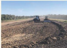
Raising a levee with new fill.
